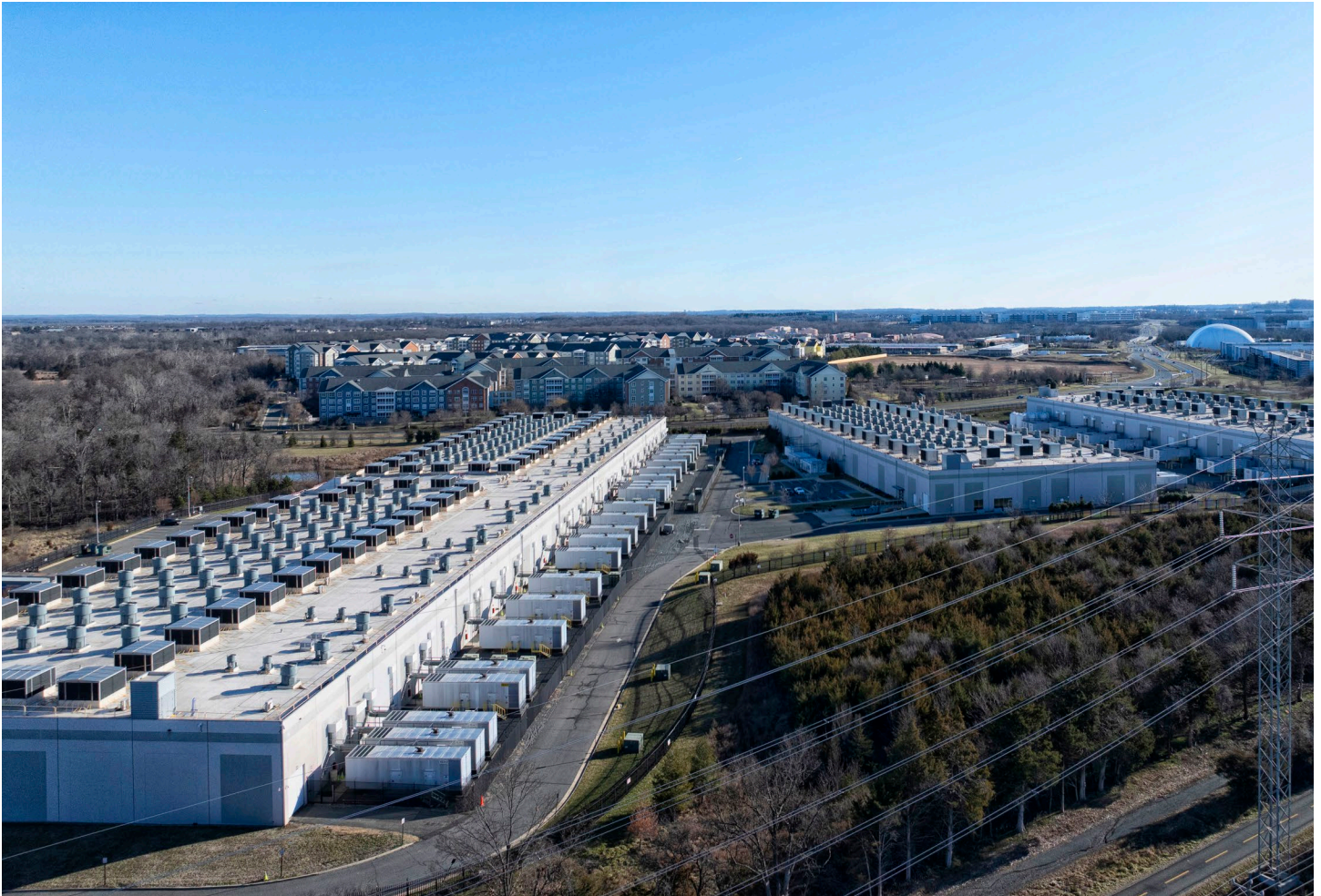
Ashburn, Virginia Data Center
